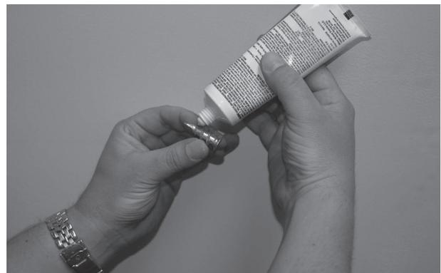
13 The left screw hole will require a drywall anchor. **Use glue** on the threads when installing this anchor to the drywall.
