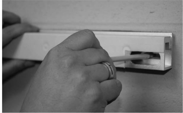
6 Level the bracket against the wall and mark the screw hole locations.
