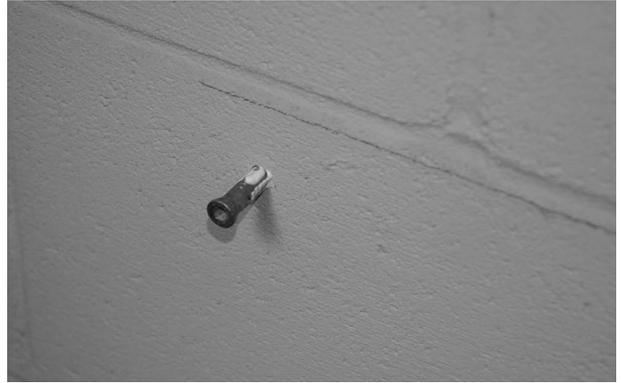
10 Push masonry anchor into wall and drive flush with hammer.
