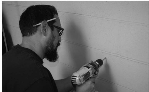
8 Drill hole for anchors using the drill / driver and 5/16 drill bit.
