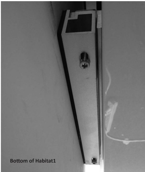
20 Secure bottom bracket with the two 50mm long cap head hardware provided from the bottom side of the bracket.
