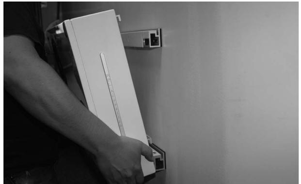
17 Connect AC cable provided to back panel of Habitat1. Lift cabinet to wall and lower onto brackets.
